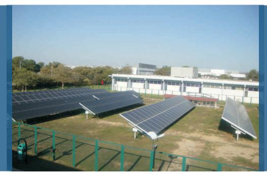
The Jaipur Plant's 40kW solar plant generates around 110 units of electricity a day.
