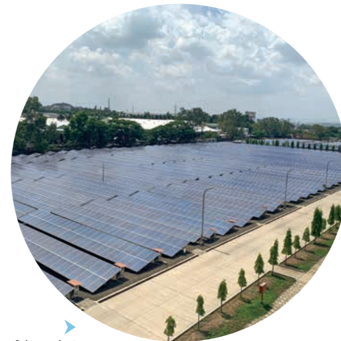
Solar panels at Nashik plant
